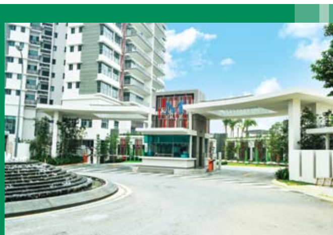
Entrance of KM1 East Condominiums at Bukit Jalil, Kuala Lumpur.
