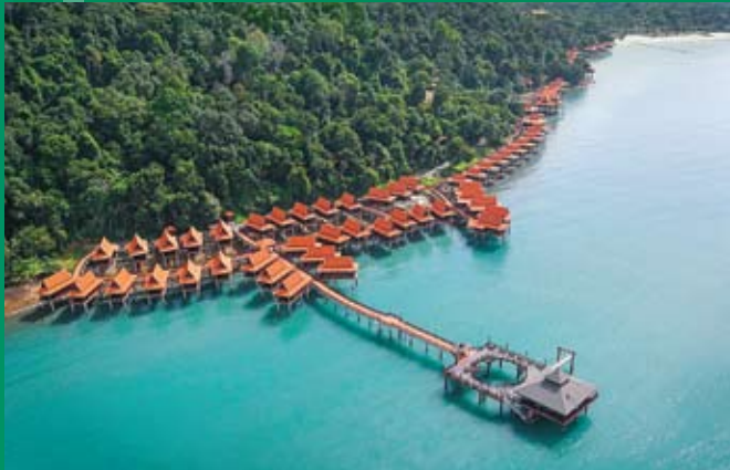
Aerial view of Berjaya Langkawi Resort, Malaysia.
