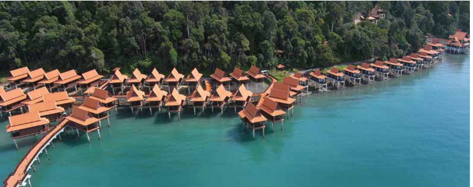
Premier Chalets on Water at Berjaya Langkawi Resort – Malaysia.
